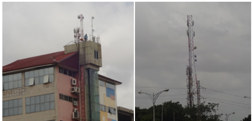
Fig. 3. (left) In the urban centres transceivers are mounted on masts high on top of buildings. (Right) In other places the mast are built to be high above trees or electricity grid
